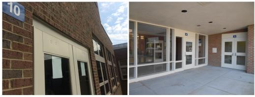
Windows: Windows should be replaced in their entirety. Steel lintels above windows are showing substantial signs of corrosion and rust. As part of a potential renovation project, it would be recommended to not only replace windows but address flashing systems within walls and window system. Water is infiltrating the buildings creating wall damage within classrooms.
